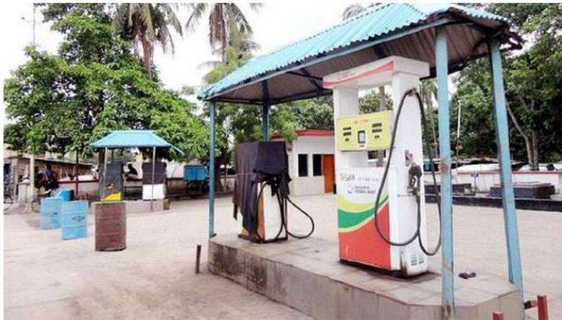
Fig. 1.1 Present Fuel Station in Bangladesh [1]
