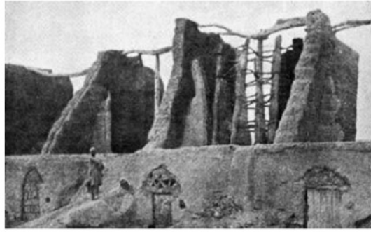
Fig 4.2: Seistan windmill (Vowles, 1932) [29]
