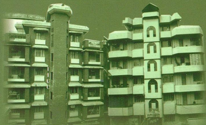
Chittagong City Campus (Academic Building 1&2)
