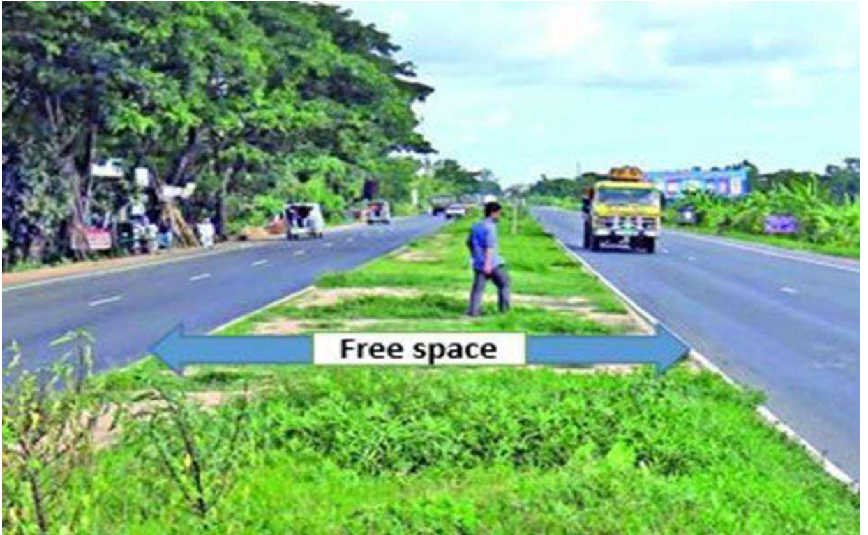
Figure1.1: Median in Roads of Dhaka- Chittagong Highway
