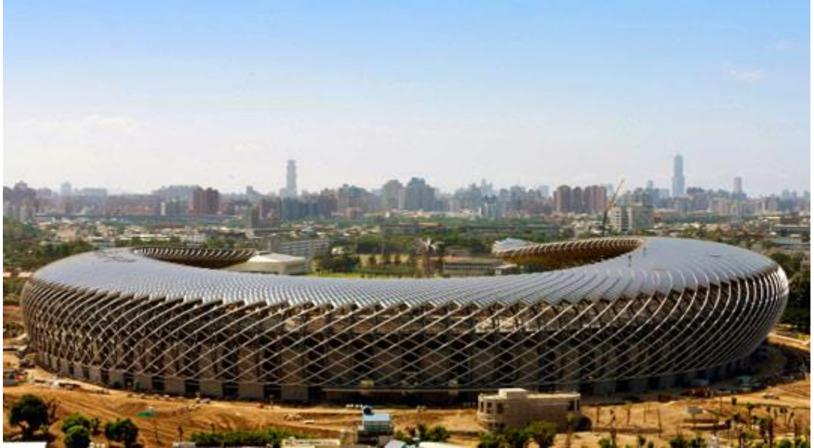
Figure 2.3: The 100% solar powered building in Taiwan[6]
