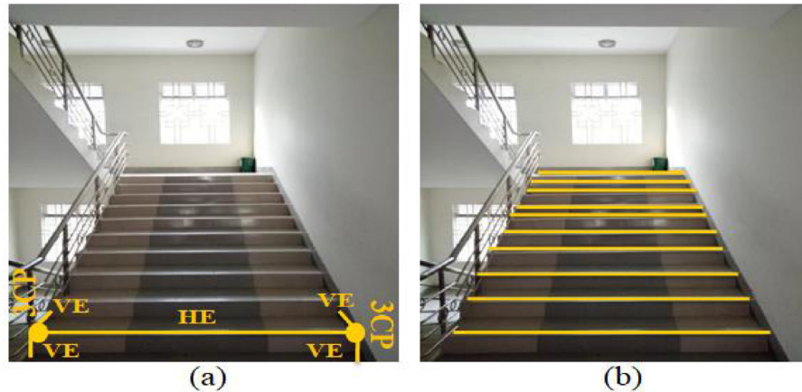
Fig. 1. Geometrical features of a stair: a) three connected point (3CP), and b) concurrent HEs are in sorted order
