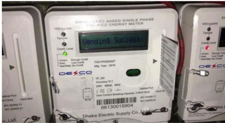
Figure 10: A digital prepaid meter being recharged by a consumer
