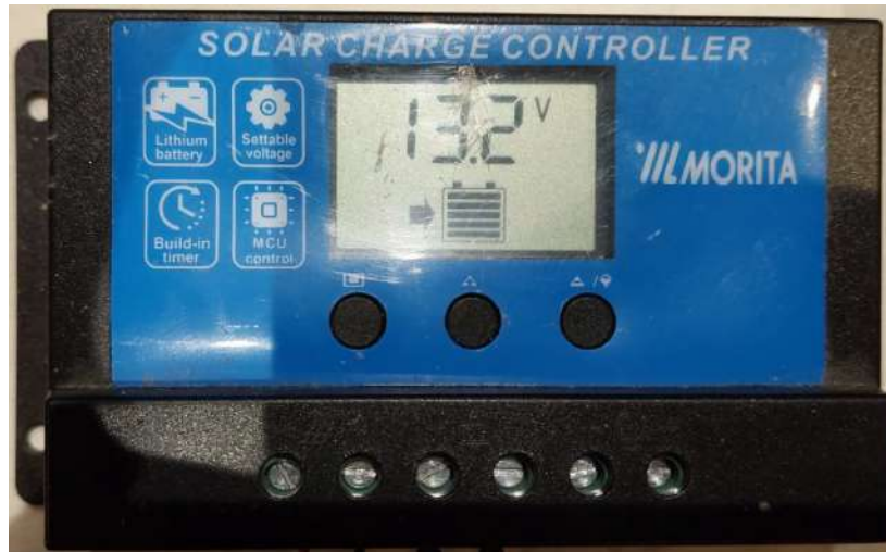
Fig. 4.16 Solar Panel Receiving Power
