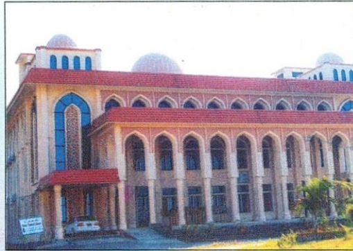
Central Library building
