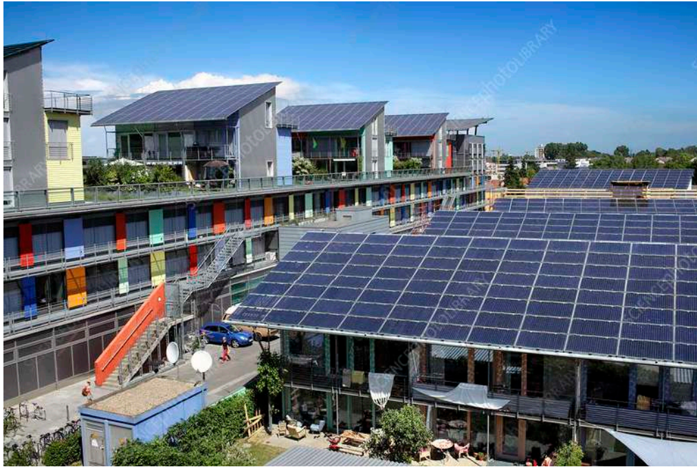
Fig. 2.4 A SHS in Germany [3]
