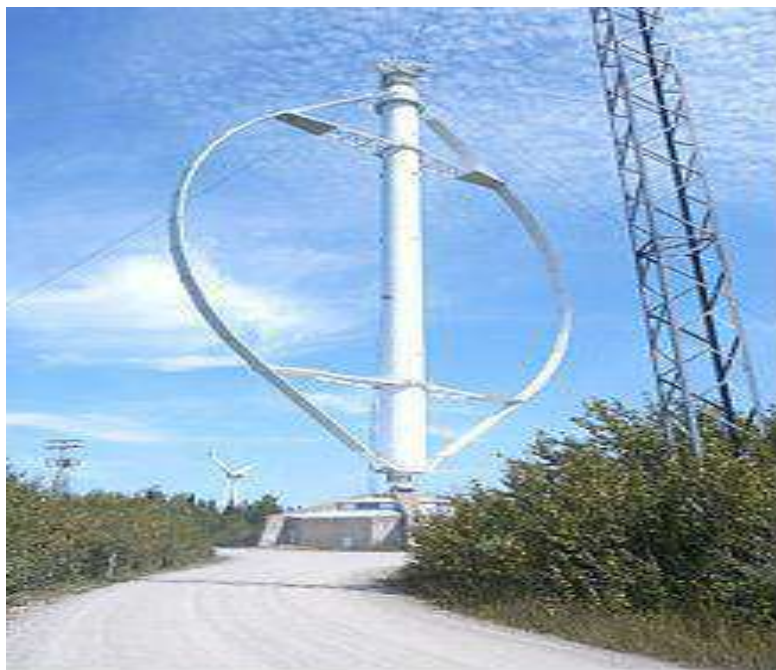
Fig. 2.3 : Vertical Axis Wind Turbine [19]
