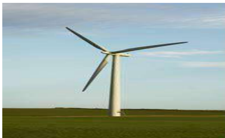
Fig. 2.2 : Horizontal Axis Wind Turbine [18].
