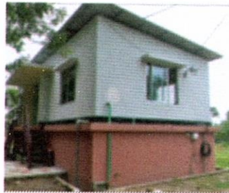
UC Water Treatment Plant
