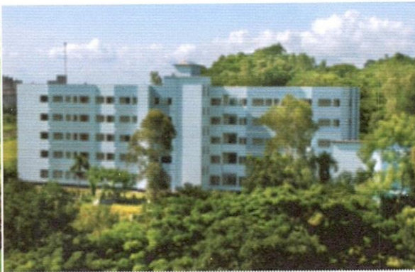
6. Science & Engineering building-1 (2nd bldg under construction)
