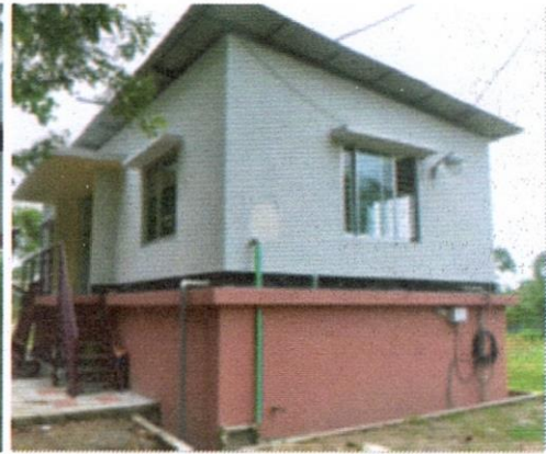
16. Water purification plant
